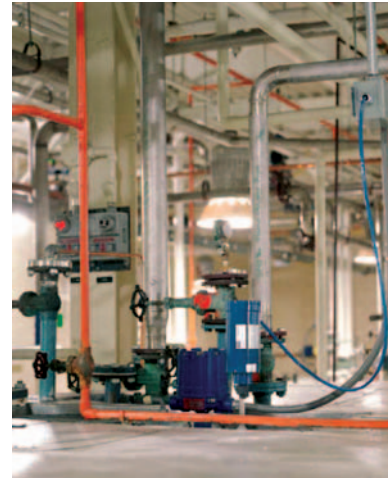
Close-up of a tank top in the wine room.
